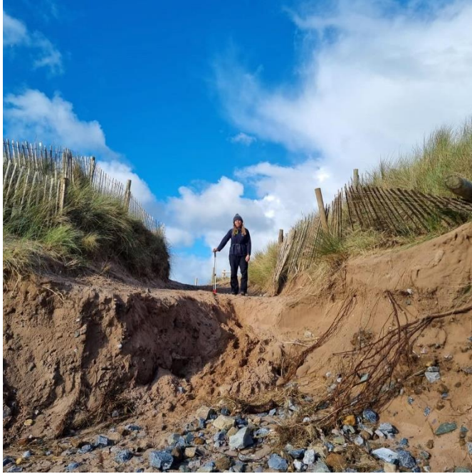
Figure 7. Storm damage/erosion at Dawlish Warren NNR.
